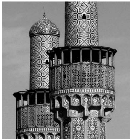
Minarette der Medrese-ye Chahar Baq / Isfahan
